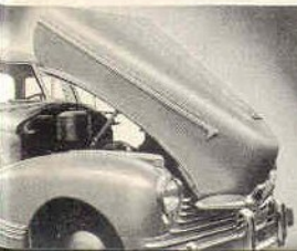
Safest hood design— hinged at the front and locked from inside.
