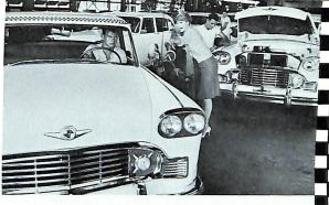
ROAD TESTED—Thorough inspections begin at the start of the assembly line and continue through every operation. After a series of final checks, the cars are critically road tested to prove that every car leaving the plant is ready to go instantly into the rigorous service demanded of a Checker car.
