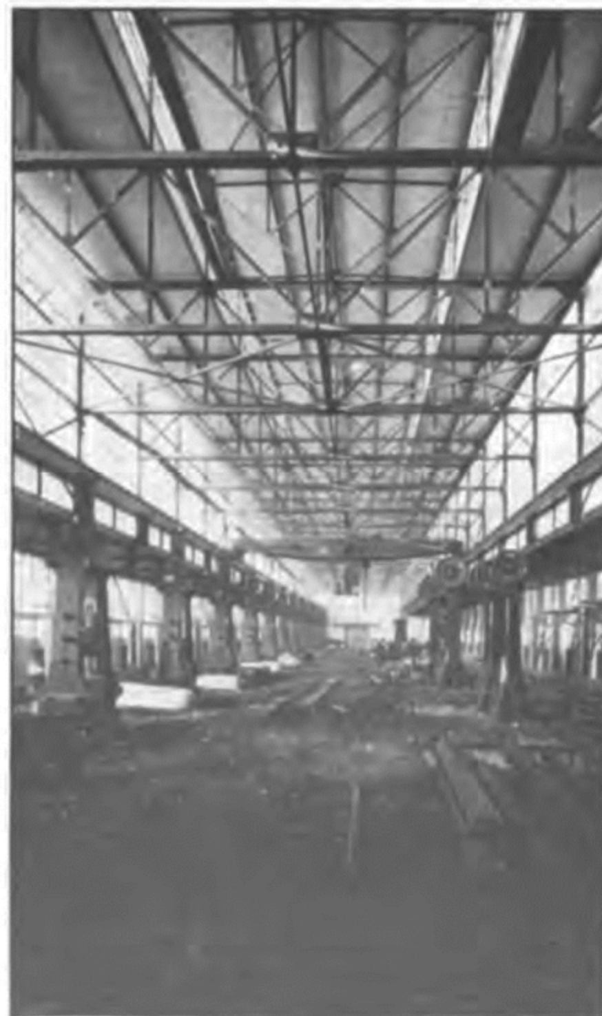
INSTALLING HAMMERS IN OUR NEW DROP FORGE PLANT
