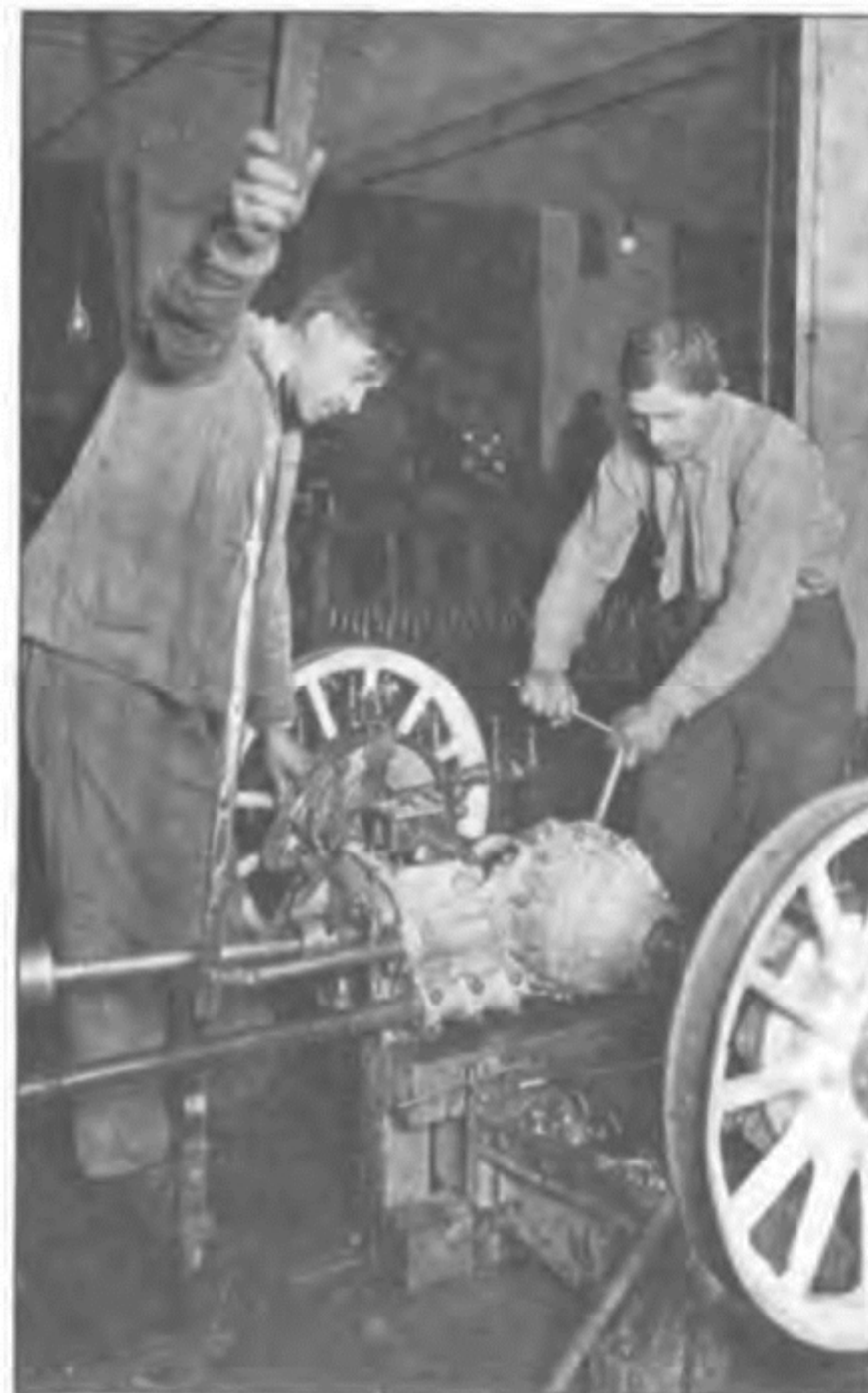
JACKING AN ASSEMBLED BRIDGE
