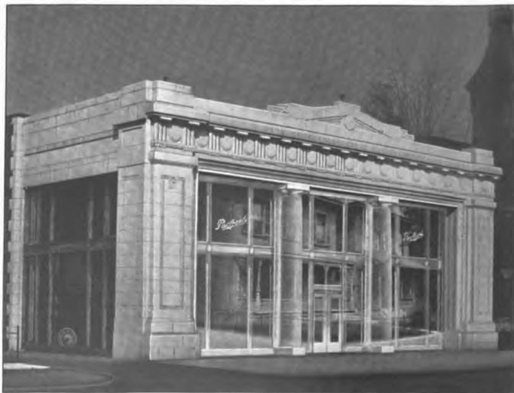
STATELY FRONT OF THE MERIDIAN AUTO COMPANY'S BUILDING IN INDIANAPOLIS. DWELLINGS OCCUPIED THE SITE LAST JULY
