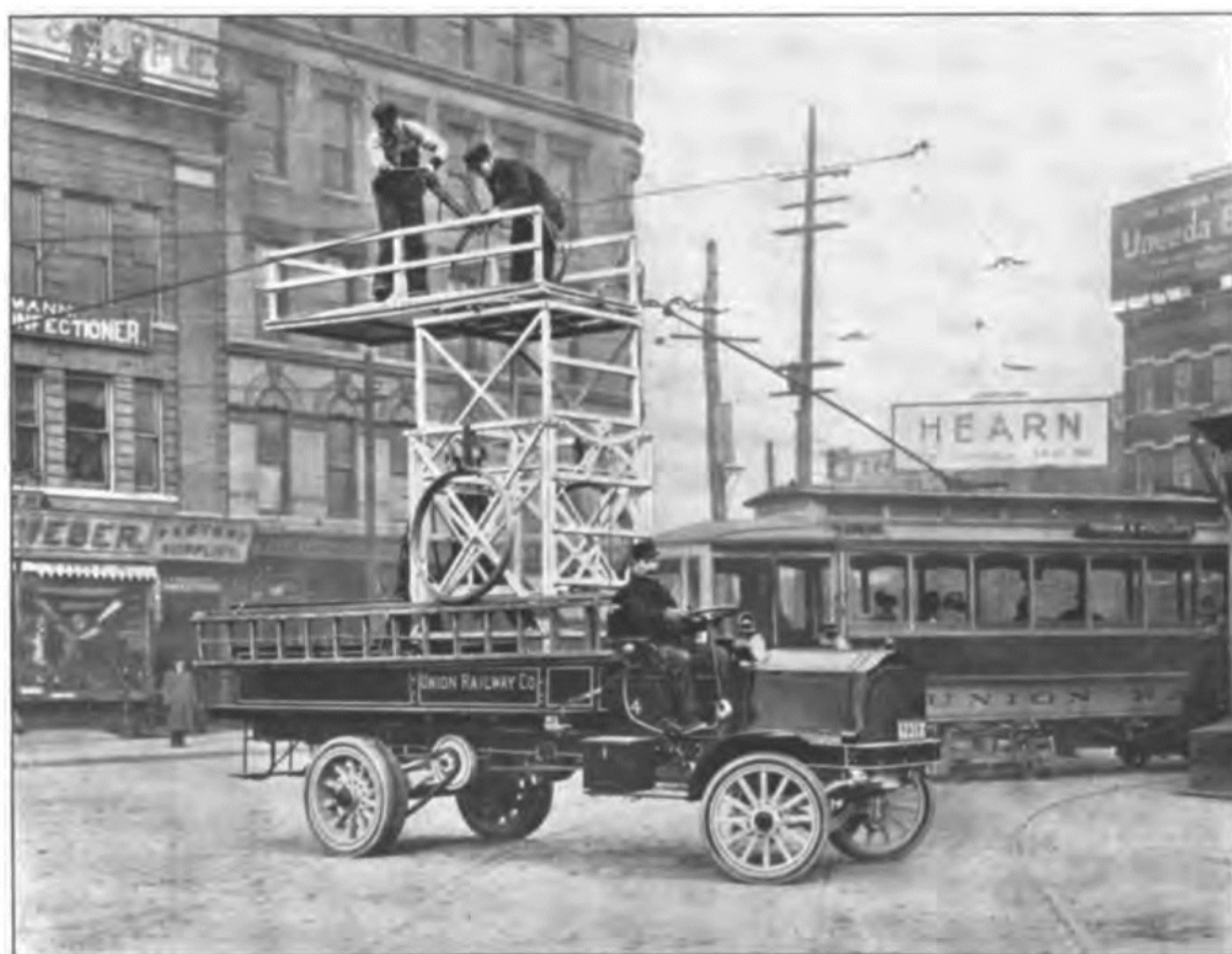
ONE OF THE QUARTETTE OF PACKARD TOWER TRUCKS IN USE IN NEW YORK
