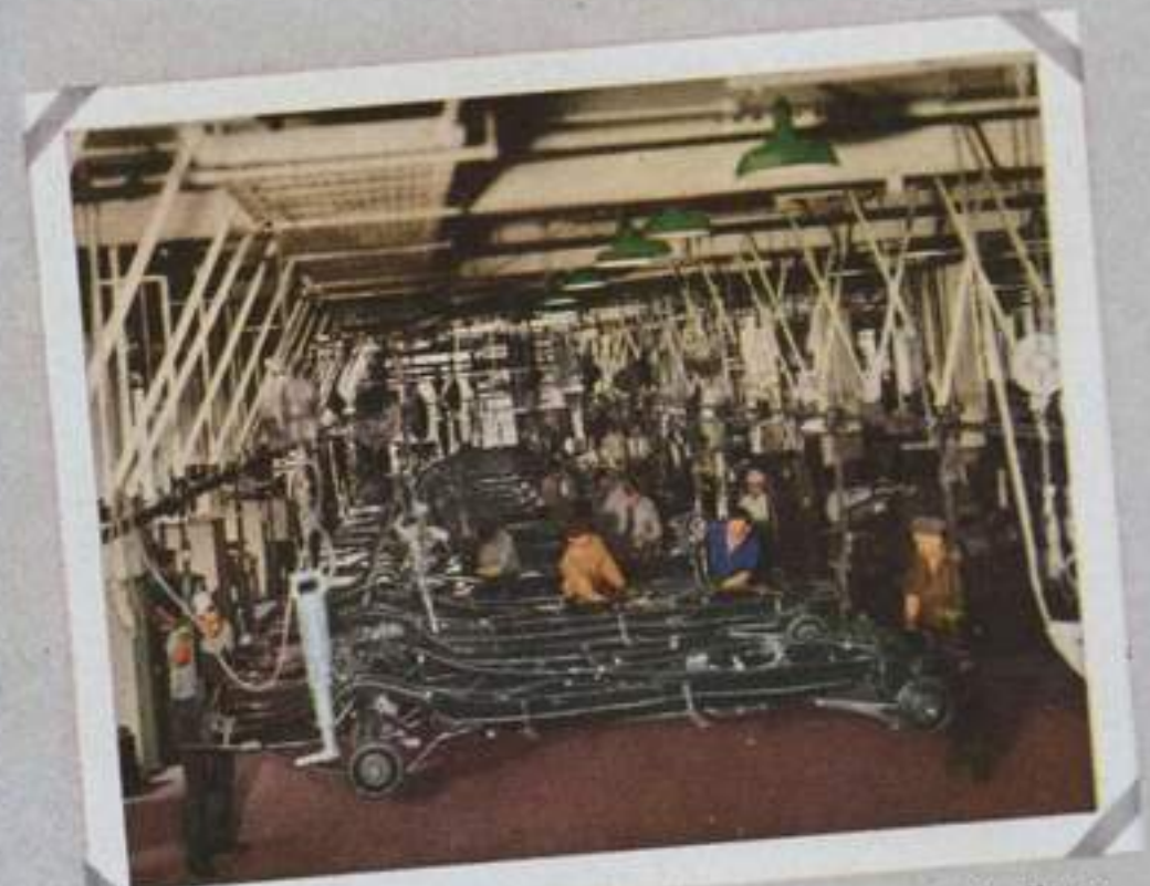
From foundry to finishing machine to testing, and finally to the chassis assembly line—Packard centralized control guards the quality of every part through every step of manufacturing.
