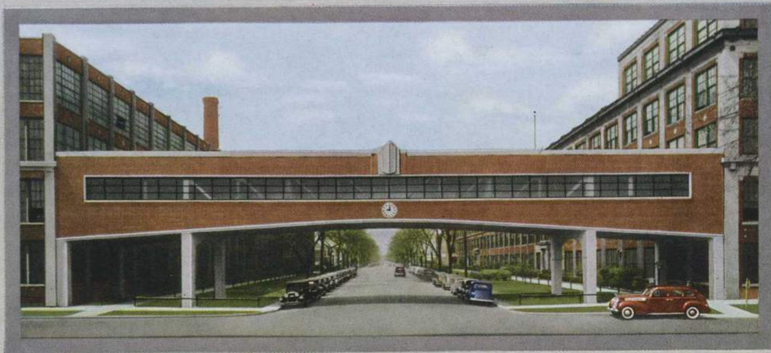
This new bridge over Detroit's Grand Boulevard connects Packard's two vast plants—symbolizes the completion of the Packard 4-year plan.
