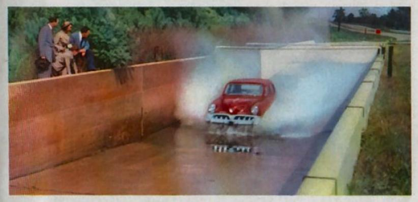
What a dousing a Studebaker can take! The ignition system has new protection against wet weather stalling. New spark plug caps act as effective "umbrellas" to prevent loss of electrical energy. Doors, windshields and trunk are sealed to keep out moisture and dust. Body insulation protects against heat or cold.
