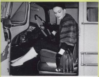
Seat adjustment when power-operated is controlled four ways with the simple operation of a single toggle switch. Where seats are hand-operated seat rises as it moves forward. An easy movement of the control handle lets the driver select the position that gives him maximum comfort, relaxation and visibility.
