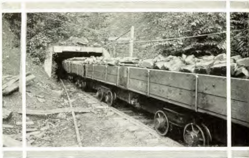
Cars of Coal Leaving Mine for Tipple, Mine No. 1, Banner Fork Operation
