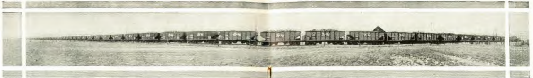
Ford Coal in Ford Coal Cars on D. T. & I. (Ford Owned) Railroad. Portion of the Equipment Utilized in the Marketing of Ford Coal
