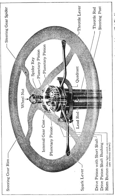
(Cut No. 1) and centre pinion. Steering Wheel, showing reduction gears meshing with the teeth of the gear case
