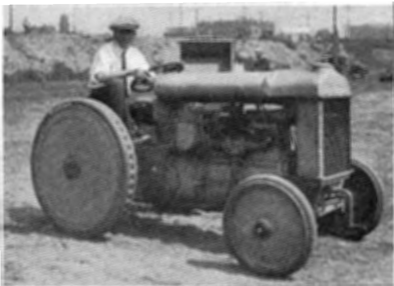
FORDSON TRACTOR WITH WHITEHEAD & KALES WHEELS AND FIRESTONE CUP CUSHION TIRES
