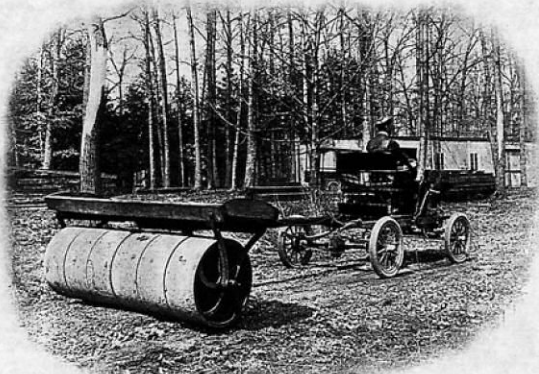
Road-Making with a MAXWELL at the Tarrytown Factory
