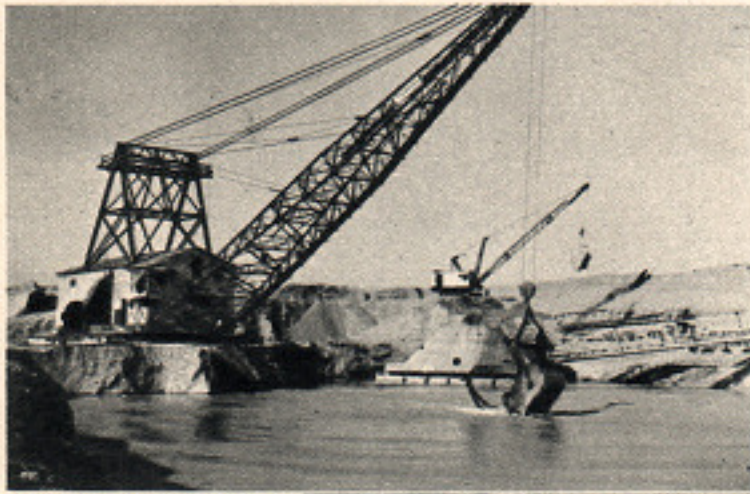
SAND AND GRAVEL . . . The production of aggregate for concrete is one of the oldest of the Kaiser industries. Established in 1914, the Kaiser sand and gravel enterprise is one of the largest of its type in the West. The plant at Radum, California, produces more than a thousand tons of concrete aggregates an hour.
