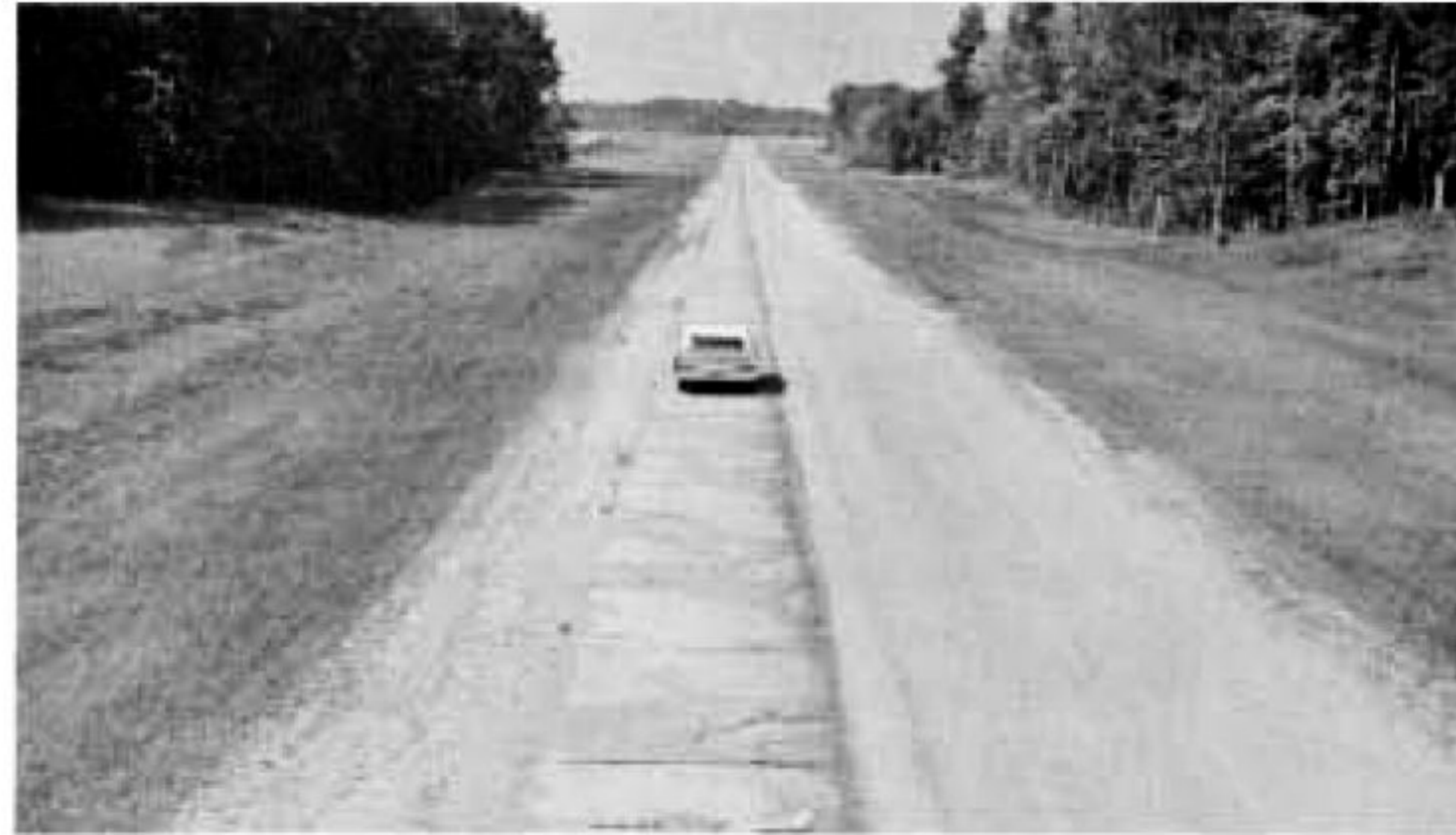
The Ride and Handling Loop, constructed in 1958, is 4 miles long and has several types of surfaces and curves for testing automobile maneuverability.
