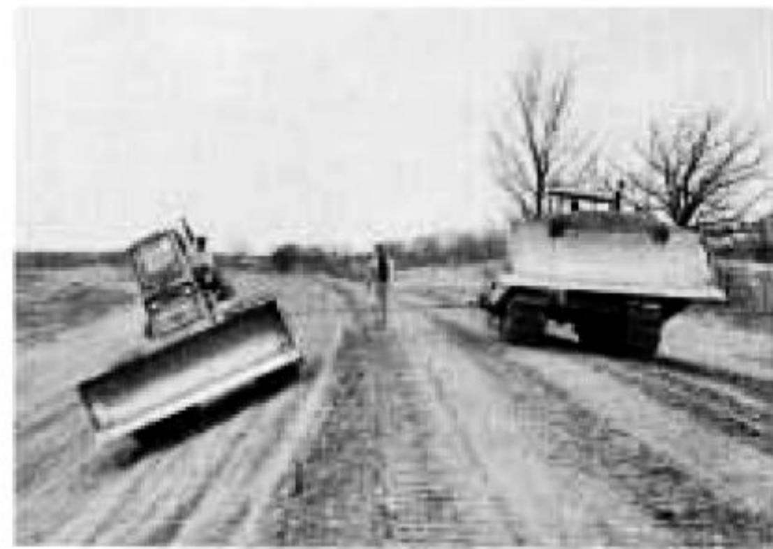
Compacting Sand Cushion
