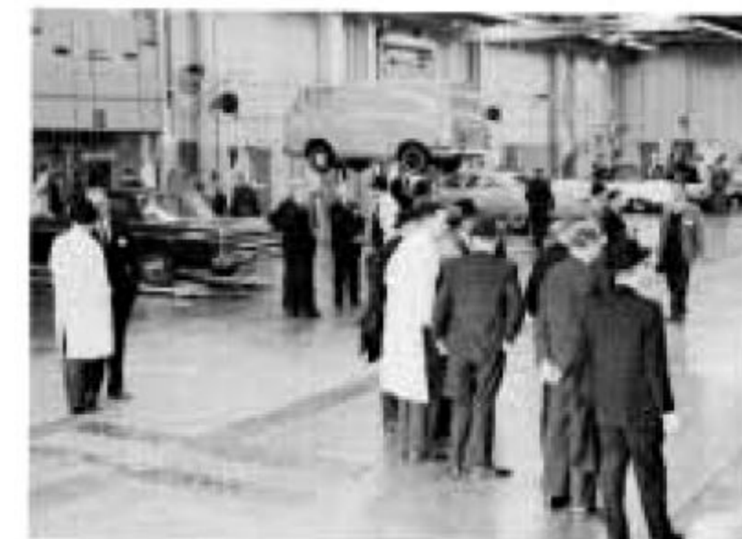
Noise and Vibration
