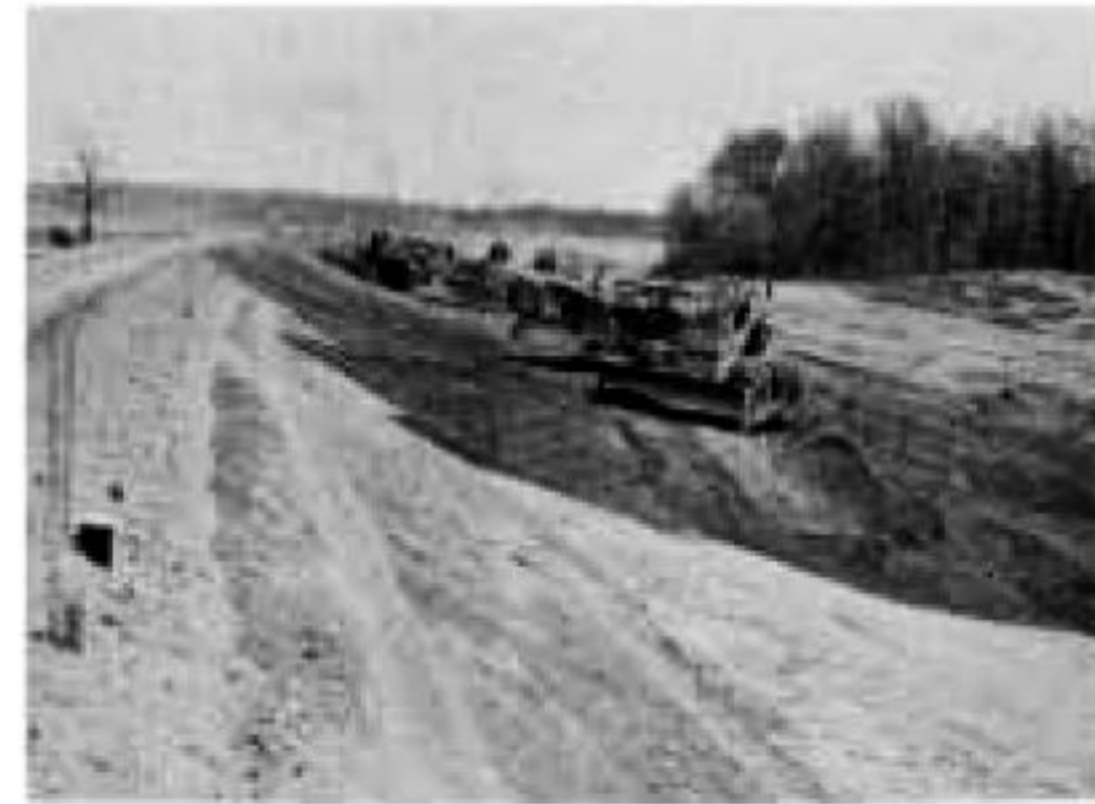
Laying Sand Cushion
