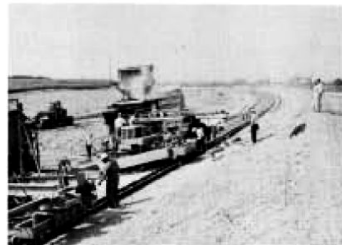
Spreading Concrete - Lane 4
