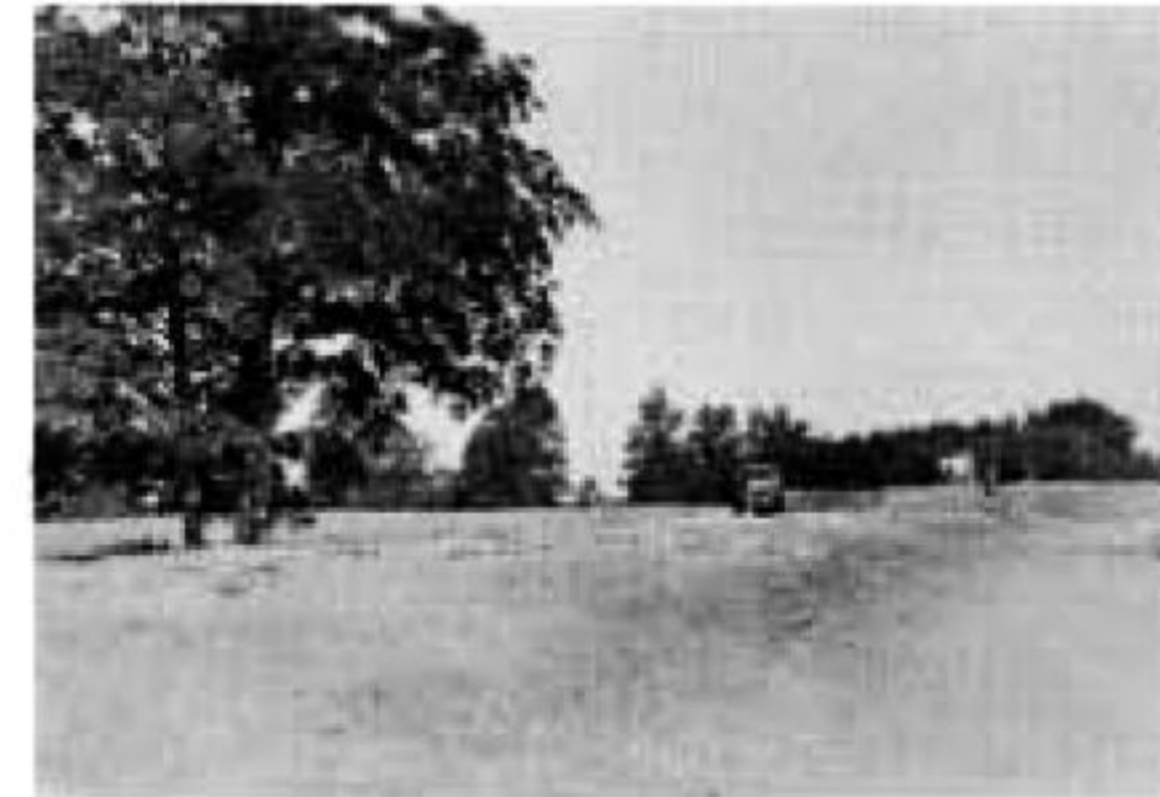
Filling Northwest Super of Oval Test Track.
