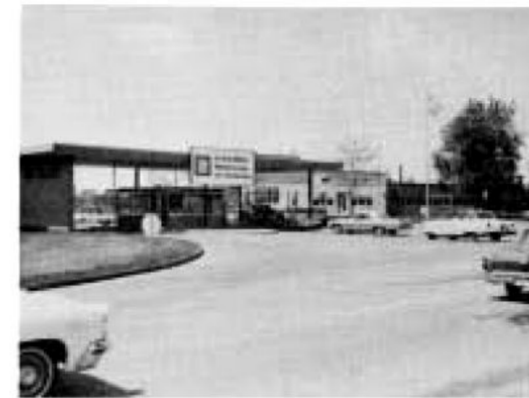
Entering the Proving Ground for "The Big Day".
