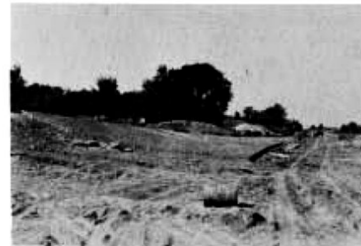
East Super Exit Transition-Gravel bed prepared for concrete surfacing.
