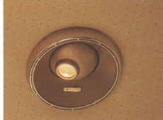
Rear compartment reading lamp.
