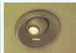
Rear compartment reading lamps.
