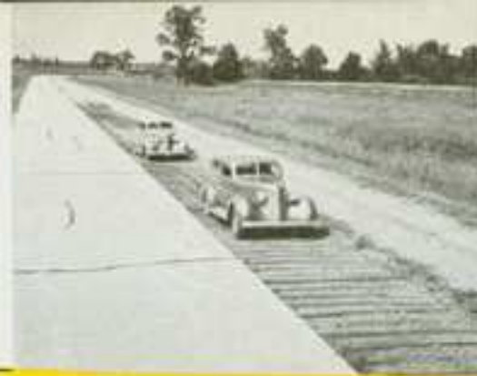
They run test cars hour-after-hour over railroad tie "roads."
