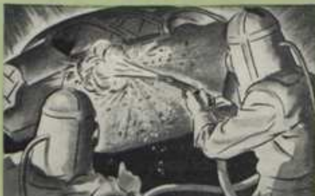
A SPECIAL sand composition is sprayed securely on the floor of each car. This forms a thick "cushion" against noise.
