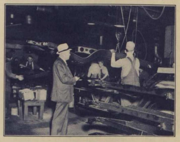
Axles and brakes are added to the frame . . . those oversized Nash brakes which give Nash cars such quick, sure stopping and long lining life.
