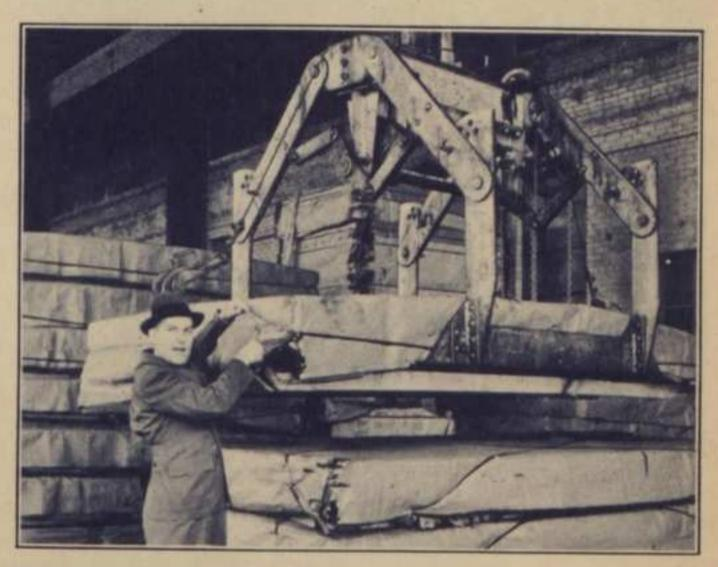
The first step, of course, is the arrival of the raw materials—particularly steel. And notice this, we insist that the smooth, polished steel sheets must come to us carefully wrapped against air and corrosive elements.
