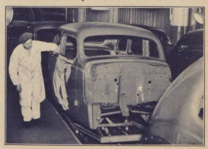
... the body shells go to one of the world's longest body assembly lines . . . 2900 feet, or more than half a mile long . . . for final body assembly. But in the meantime
