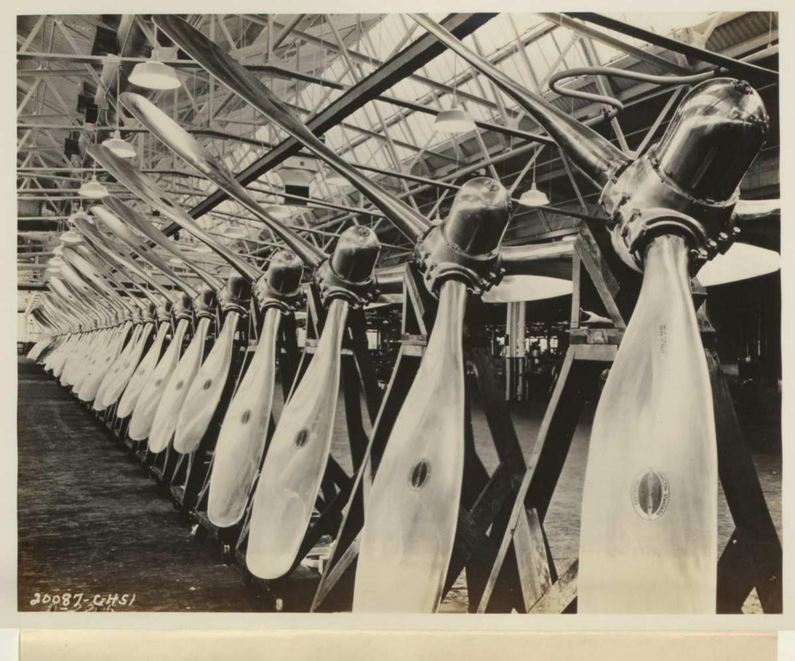
Newest development in aircraft controlled-pitch propellers is the Hamilton Standard three-bladed hydromatic propeller, which Nash-Kelvinator Corporation will manufacture as part of its more than \$100,000,000 in National Defense Contracts. A former auto plant in Lansing, Mich., is being converted into a modern aircraft factory for this purpose.
