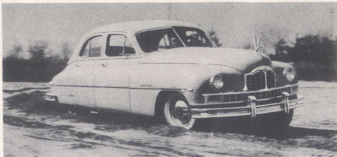
Durability test: Pull out of deep sand as shown without chatter.
