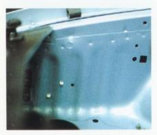
Convolutions stamped into the unibody are intended to help the body absorb impact forces in a controlled manner.
