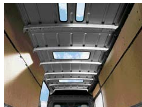
Skylights in load compartment.
