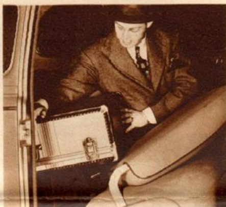
Coupe trunk is accessible from inside! This innovation, as introduced in the Champion, is appreciated by salesmen and other drivers in stormy weather. Sample cases or other articles may be reached merely by tilting the seat forward. In addition to the accessible trunk space, there is ample room for brief cases on the wide shelf above the seat. Studebaker has been notable for the roominess of its trunks—and this Champion's space is remarkable.
